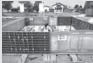
Wall Formwork
