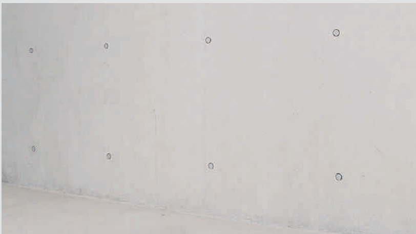
Concrete cones with shadow joint glued in place.
