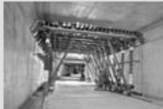
Tunnel Formwork
