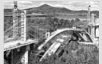
Bridge Formwork
