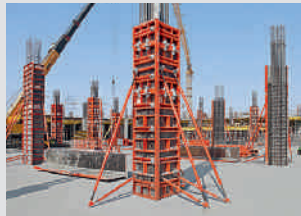
Column Formwork
