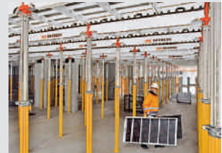
Slab Formwork
