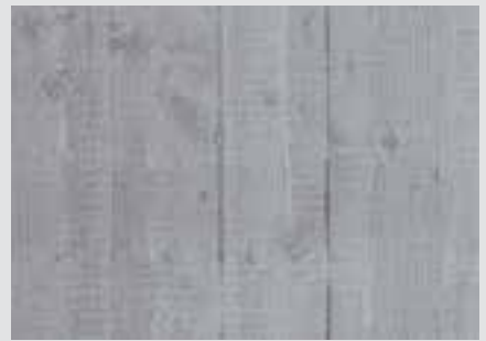
Girder formwork with individual boards
