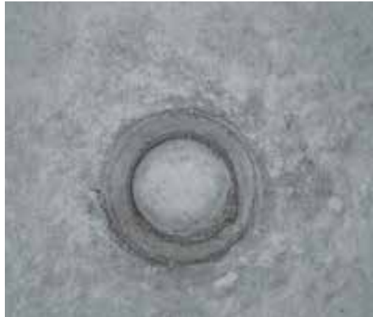
Unused tie points in the large panel; sealed with plastic plugs
