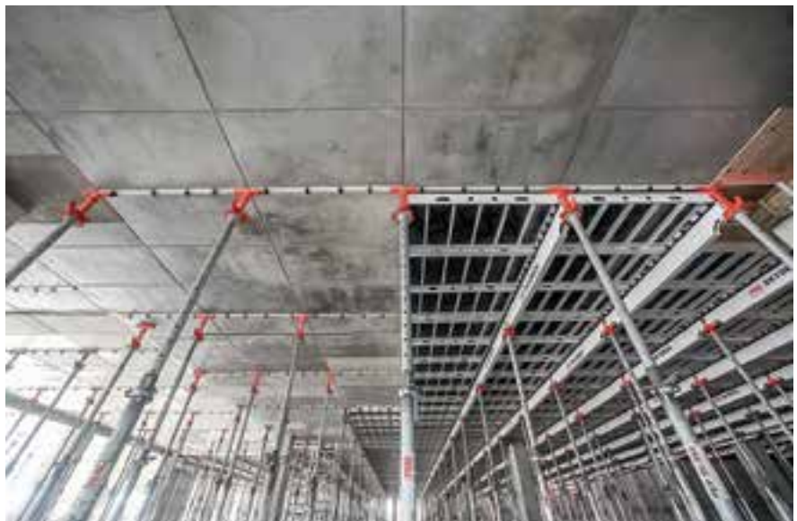
Slab soffit formed using SKYDECK Dropheads. Grid: 1.50 x 2.30 m
