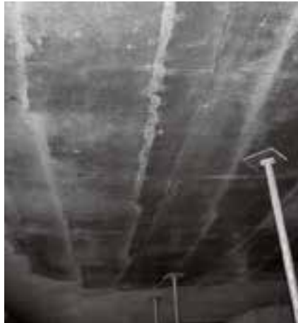
Visible "continuous spacer". "Continuous spacer" laid with flat side on formwork.
