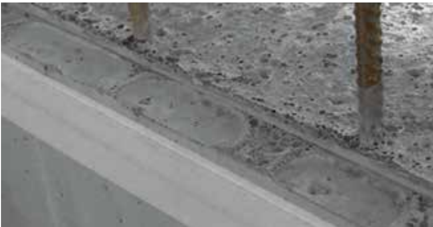
Air bubbles under the height indicating strip. Underside of the height indicating strip not chamfered.
