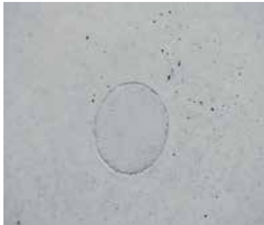
MAXIMO tie point sealed with a fibre cement plug
