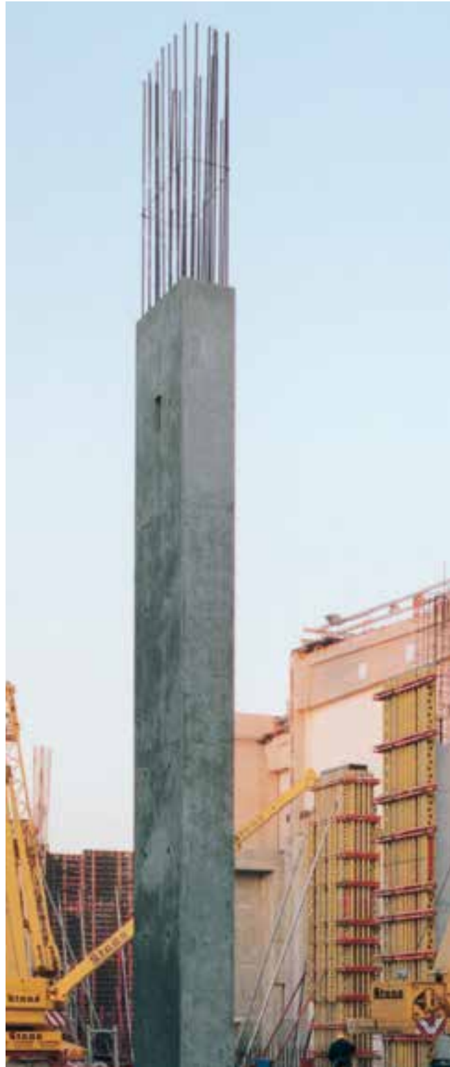
Column formed with VARIO Column Formwork
