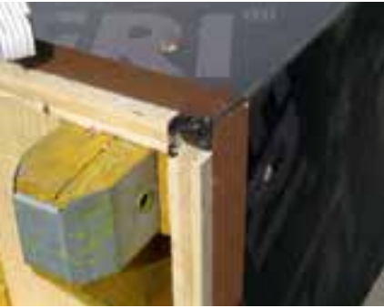
Mitre joint with silicone grouting
