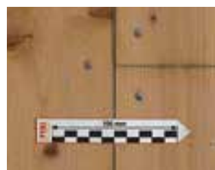
Example of fixing: Nails
