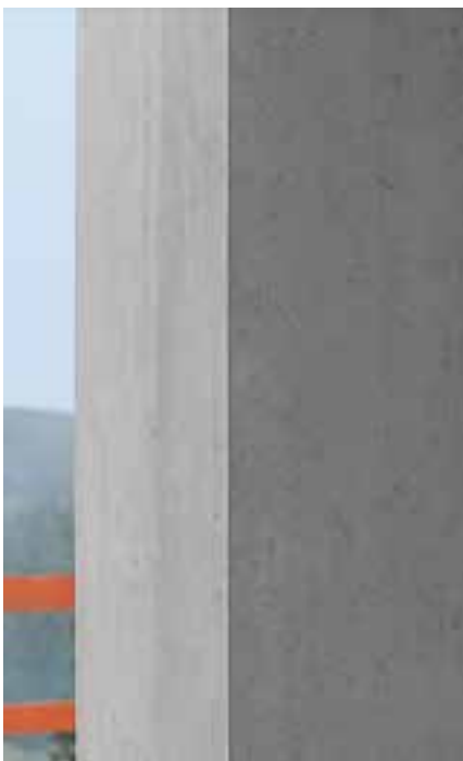
Column formed with RAPID Column Formwork, edges bevelled through the use of chamfer strips
