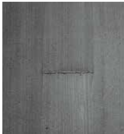
Surface from boarded formwork: self-compacting concrete
