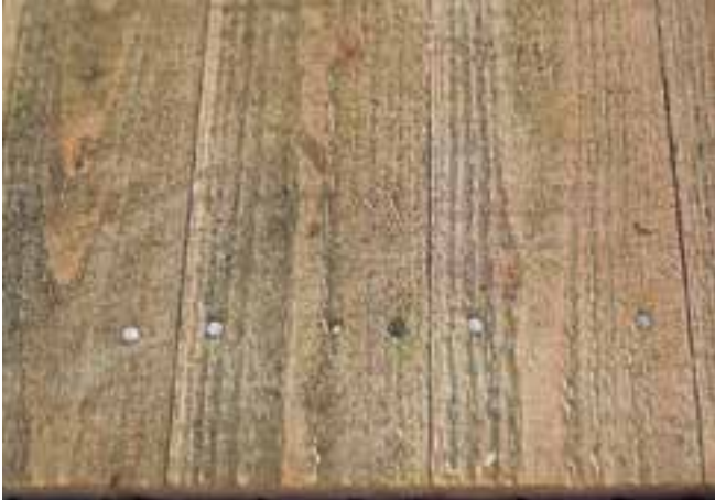
Formlining: rough-sawn boards, rough, nailed.
