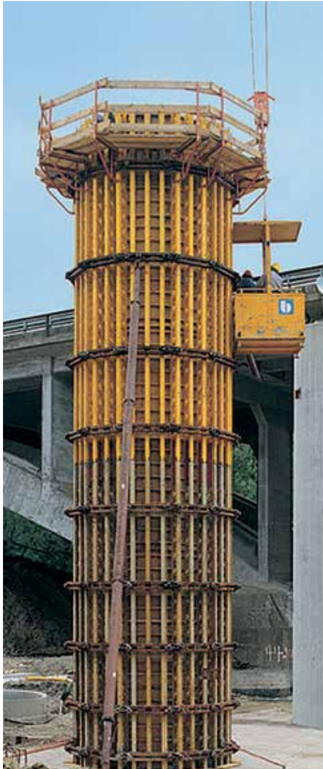
Column formed with articulated waler formwork
