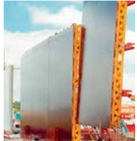
A uniformly thin application on the formlining is recognizable by a matt gloss finish.
