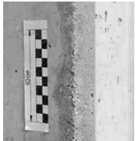
Bleeding in the corner area and dark discoloration. Wooden chamfer strip and nailed to stopend formwork.
