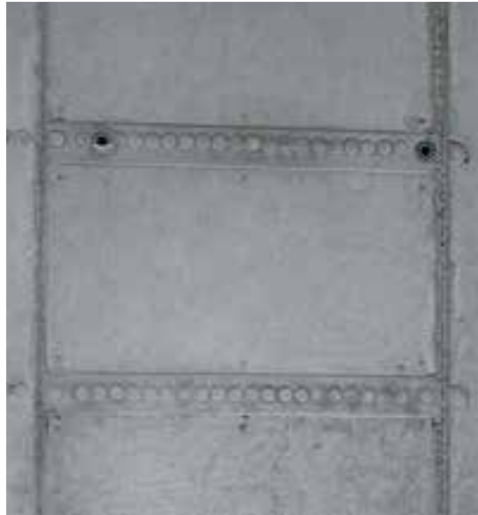
Concrete finish using a multi-purpose panel
