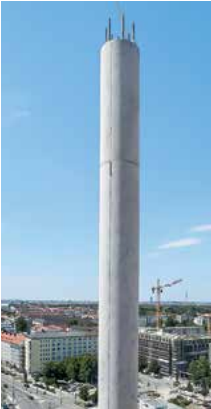
Column formed with VARIO Column Formwork
