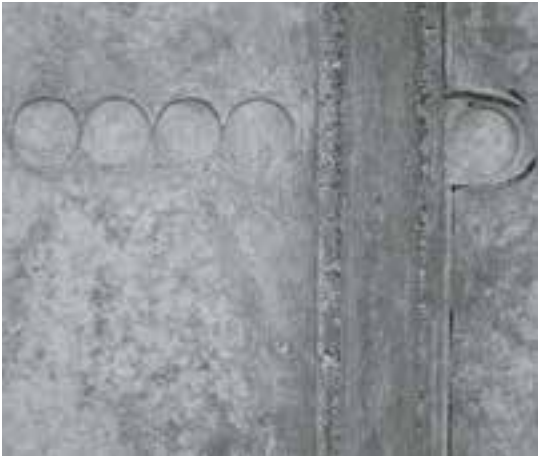
Articulated corner, steel filler and standard panel details; tie points sealed by means of plastic plugs
