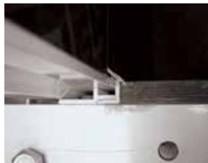
Corner details: RAPID Column Formwork with 30 mm thick formlining without chamfer strips for sharp-edged columns.
