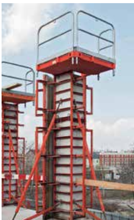
Column formed with QUATTRO, the formwork features a double height extension
