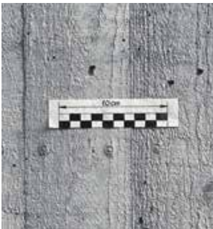
Surface texture through boarded formwork: Vibrated concrete
