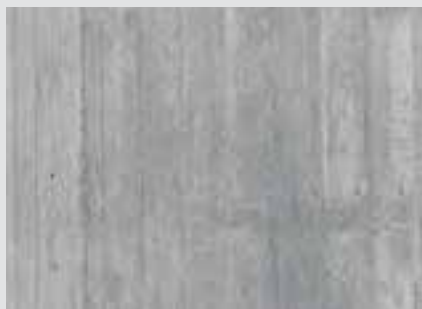
Element joint impression of girder formwork with boards as formlining
