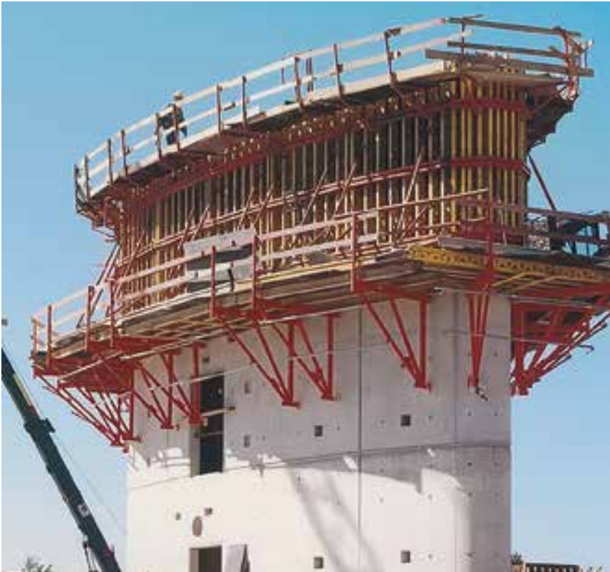
Stairwell walls, ground plan with changing radii. Formed with VARIO elements and double-layered profiled timber
