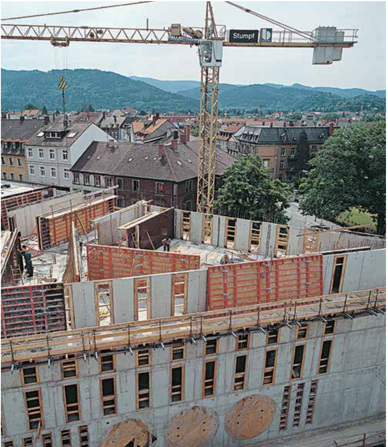
Wall constructed with TRIO Structure
