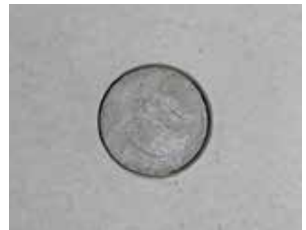
Plugged with flush-fitted concrete cone
