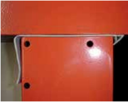
Attaching chamfer strips in box outs and stopend formwork
