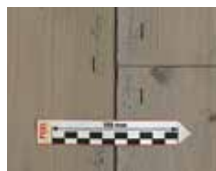
Example of fixing: staples
