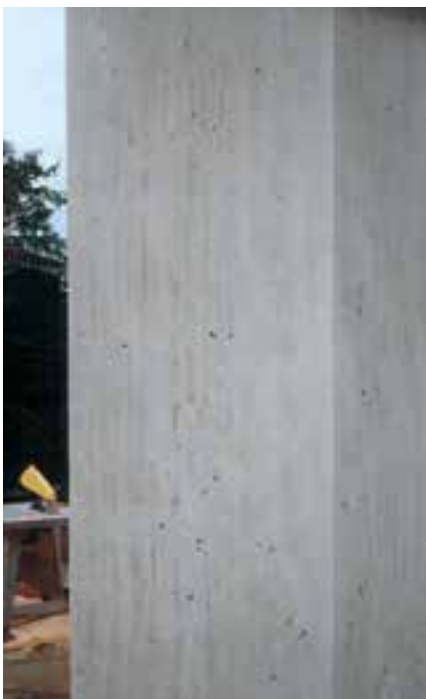
Corner details: RAPID Column Formwork with 30 mm thick formlining without chamfer strips for sharp-edged columns.
