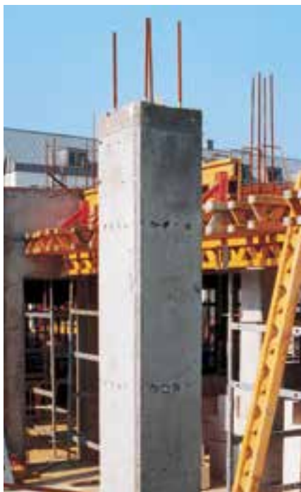
Column formed with TRIO Column Formwork
