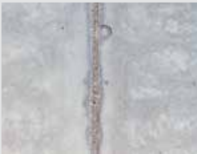
Element joint impression of panel formwork
