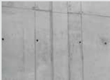
Element joint impression of panel formwork
