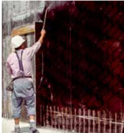
Uniform, thin release agent application is not possible in this way.
