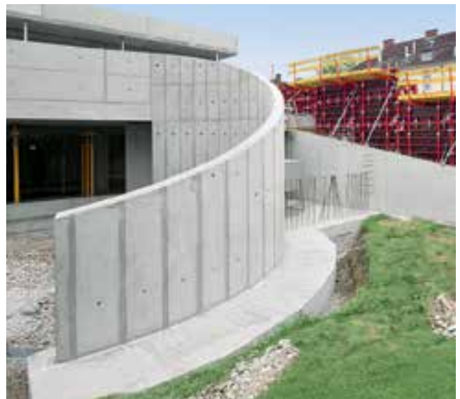
Curved wall formed with MAXIMO elements with trapezoidal strips inserted in the joints.
