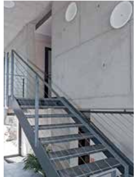
Horizontal formwork panels, offset by half a width
