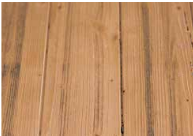
Formlining: 3-ply plywood, brushed surface, coated, with milled grooves.
