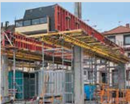
With the ST 100, heavy beams can be concreted in advance. This can be done very quickly as the ST 100 very often does not require any diagonals.
