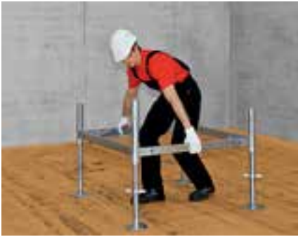
To set up the Base-Head Frame adjust base spindles to required height and level accordingly.
