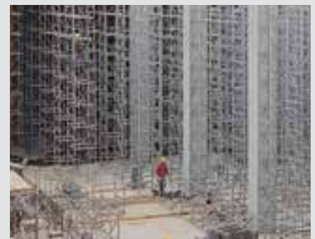
For larger heights, the ST 100 is horizontally pre-assembled. The diagonal bracing ensures the structure is tightly connected for transport with the crane.
