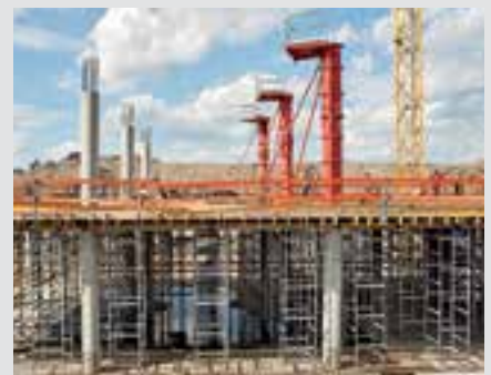
Even without diagonals, the PERI Stacking Tower is capable of carrying loads. (Take type test into consideration).
