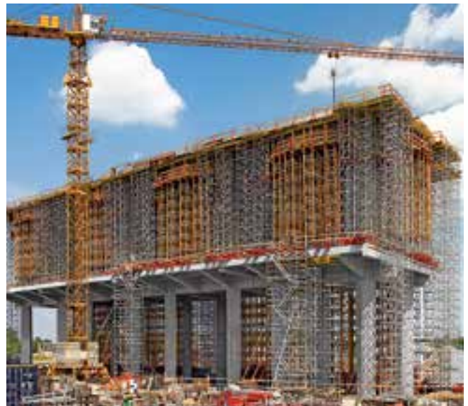
The modular MULTIPROP system and ST 100 Stacking Towers, ideally combined. Rentable SRZ and SRU Steel Walers from the VARIO wall formwork product range were used for load distribution.
