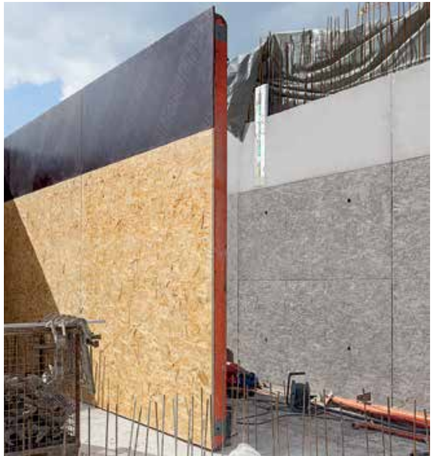
With TRIO Structure, SB 3 architectural concrete requirements are fully met. The OSB sheets and FinPly formlining were neatly screwed on at the rear.
