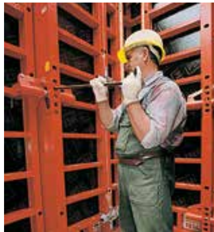
When striking, the crane slings are attached to all four Shaft Panels and the formwork panel is brought into the striking position by means of levering.
