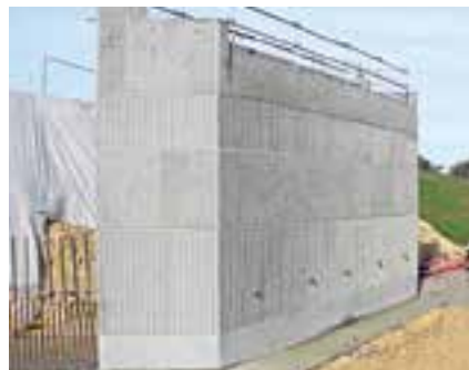
With TRIO Structure, SB 3 architectural concrete requirements are fully met. The OSB sheets and FinPly formlining were neatly screwed on at the rear.
