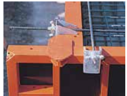
The Top Tie Bracket allows grid-independent anchoring outside of the panel. As a result, it is used for foundations and extensions.
