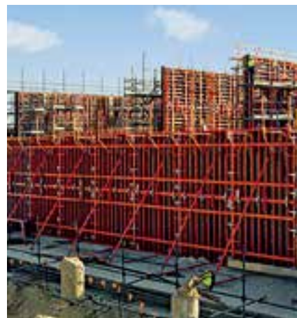
TRIO can be extended up to heights of 5.40 m in 30 cm increments. For larger heights, a compensation water is also used.
