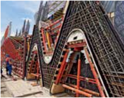
Prosta Tower, Warsaw, Poland
