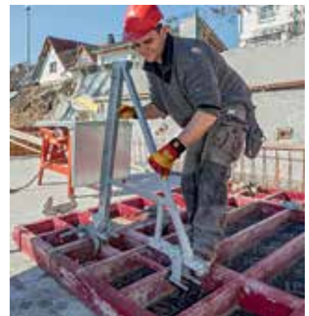
The working platforms are mounted on the element of the corresponding width and also remain attached to the formwork during temporary storage.
