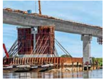
Vistula Bridge, Kwidzyn, Poland
