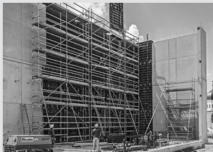
Working scaffolds construction
