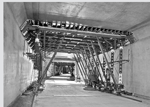
Tunnel formwork
