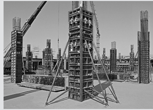
Column formwork
