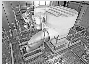
Working scaffolds industry
