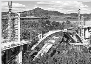
Bridge formwork
