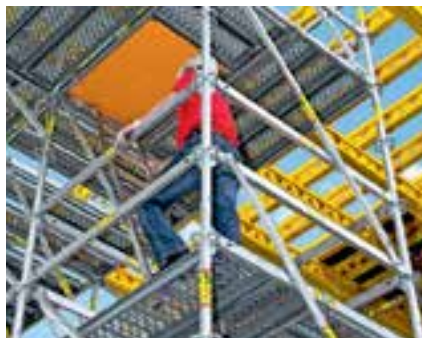
As access to the upper working platforms on shoring towers, hatches with separate ladders can also be used in bays with lengths of only 1.50 m.
