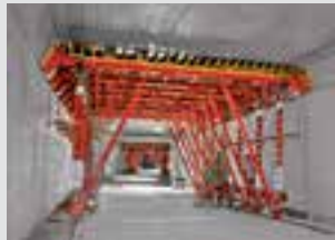
Tunnel Formwork
