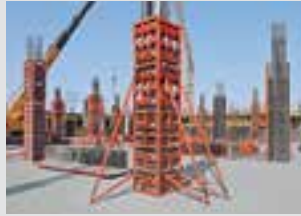
Column Formwork
