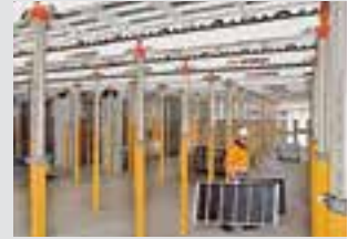
Slab Formwork
