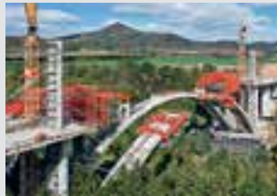
Bridge Formwork
