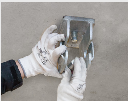
Step 4 Fixing the Suspension Head VGK with the nut M24
