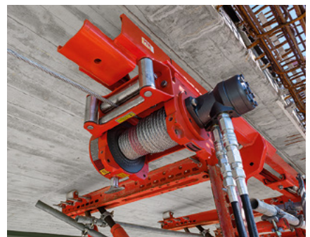
The units could be moved quickly thanks to an integrated cable winch.
