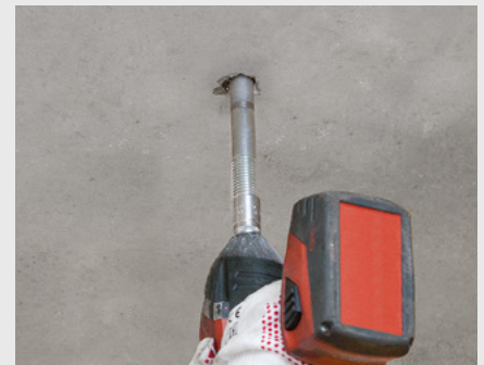
Step 3 Screw in the refurbishment anchor by means of an impact wrench
