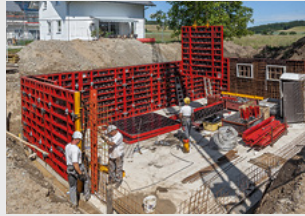
Wall Formwork
