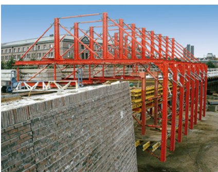
The VGW can be adapted to accommodate a wide range of cantilevered parapet geometries.
