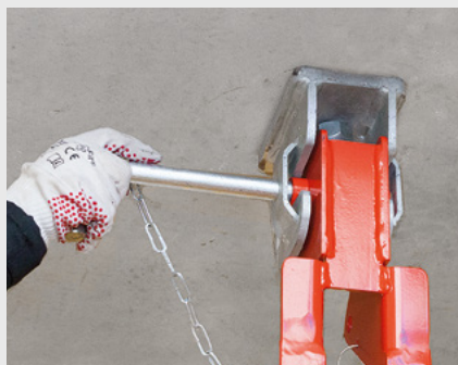
Step 5 Fixing the VGK with bolts
