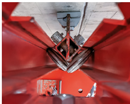
The VARIOKIT Cantilevered Parapet Track was suspended by means of rails and Roller Units from the underside of the bridge cantilever – at an identical position to the moving procedure and concreting.
