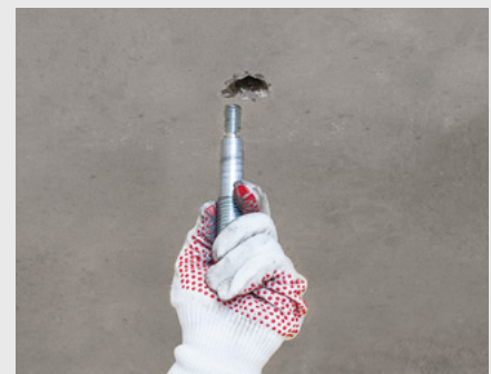
After dismantling the console bracket Remove the reusable connecting element
