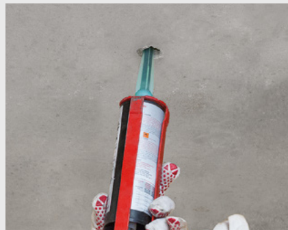
Step 2 Inject the composite mortar
